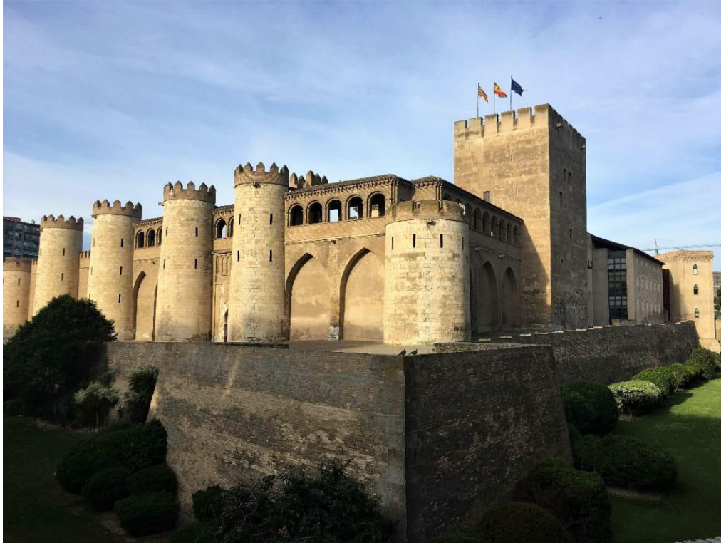
Fig. 1 General exterior view of the Aljafería Palace with its 'torre del Homenaje' (donjon). Photo: Juan Carlos Lozano López
