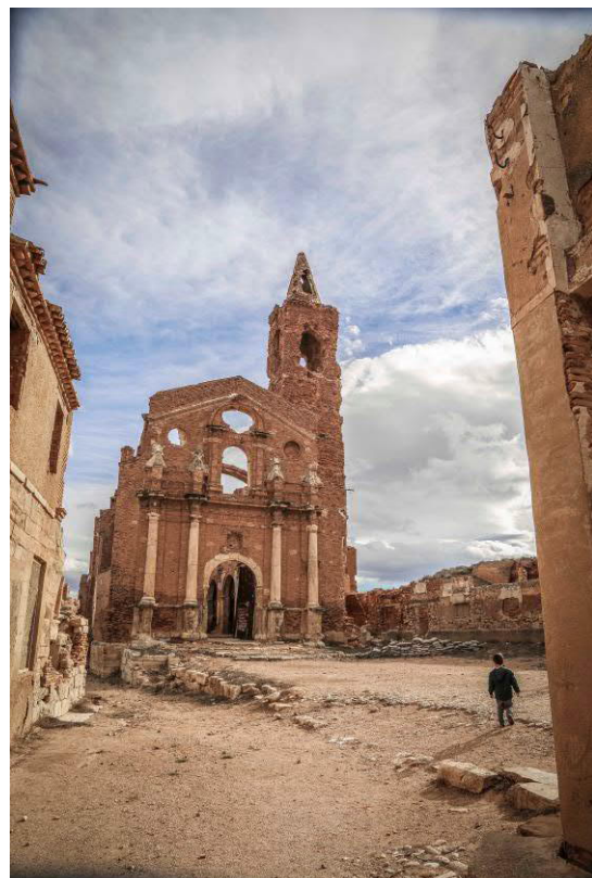
Fig. 2b Partial view of the ruins (Church of St. Martin from Tours), Belchite, Zaragoza, Spain. Photo: Ascensión Hernández Martínez
