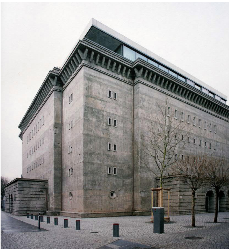
Fig. 6 Former bunker housing the Boros Collection, Berlin, Germany. Photo: Ascensión Hernández Martínez
